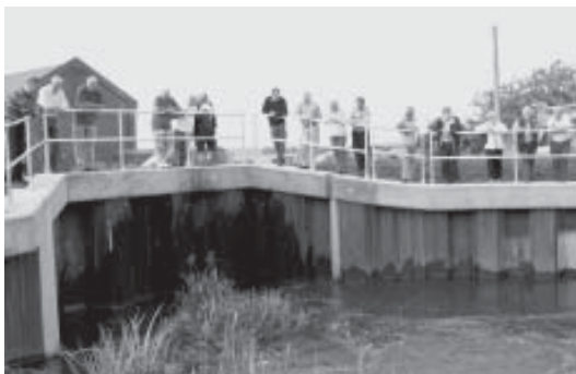
HCS members at pump outlet Swallows nest under top cladding
