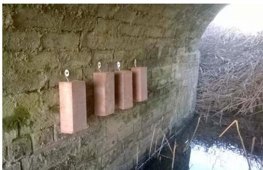
*Bat bricks fitted in a Churchfield & Plawfield IDB culvert, (image WP\_20150217\_002).*
