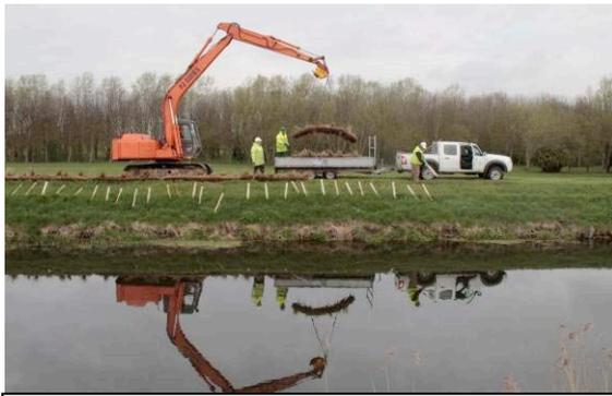
*Above, coir rolls being installed on the Old River Nene near Ramsey IDB, (image MG\_6211).*
